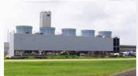
MARSHALL SPACE FLIGHT CENTER CENTRAL ENERGY PLANT
