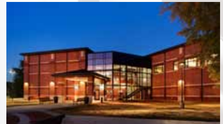
REDSTONE ARSENAL MECHANICAL SYSTEM
