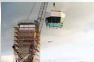
AIR TRAFFIC CONTROL TOWER FAB AND INSTALL
